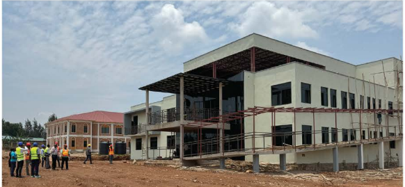
Existing Buildings on Site
