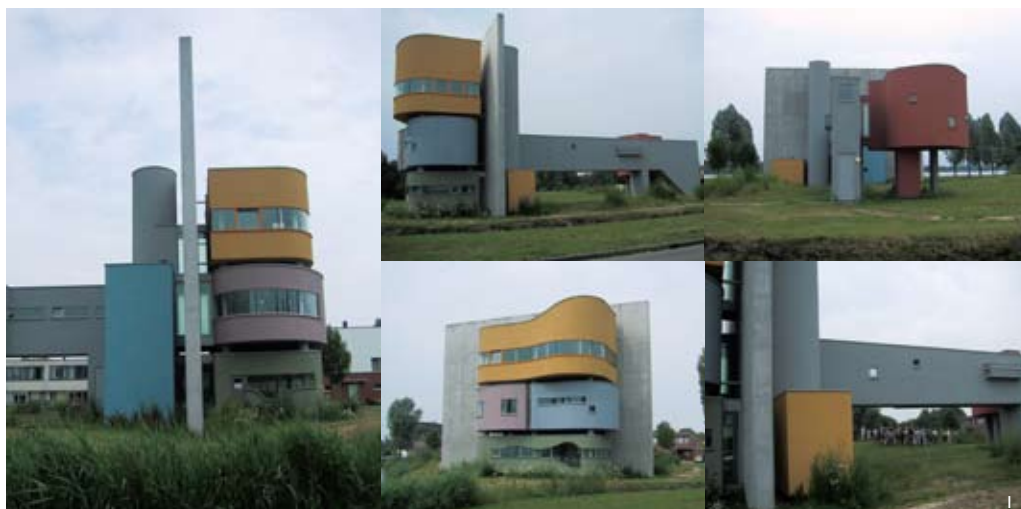
1. 墙宅之二室外 2. 墙宅之二平面图 1. Exterior views of Wall House 2 2. Plans of Wall House 2
